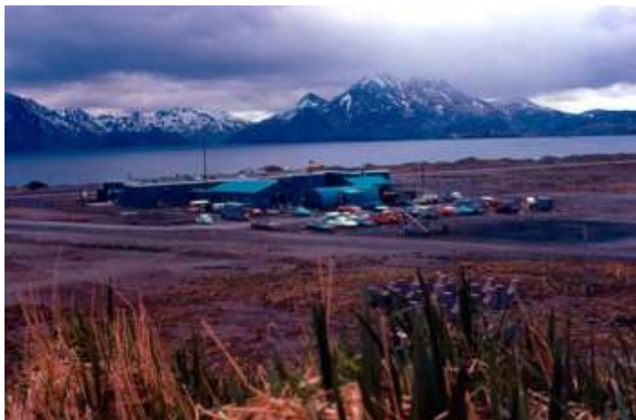
Naval Facility Adak
