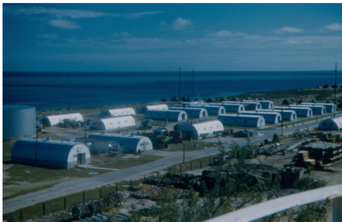
Seabees arrive to rebuild the NavFac.
