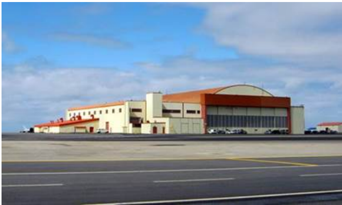
Hangar 831 completely reconstructed
